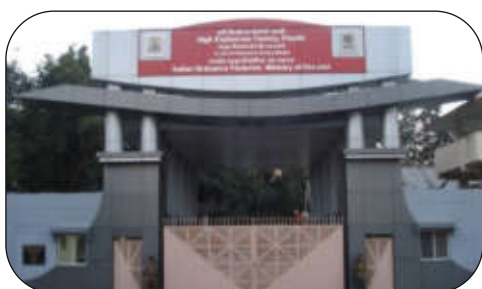
High Explosive Factory Khadki (HEF)
